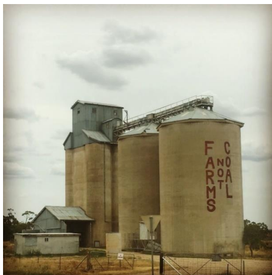
Figure 3. Silo, Liverpool Plains, NSW
