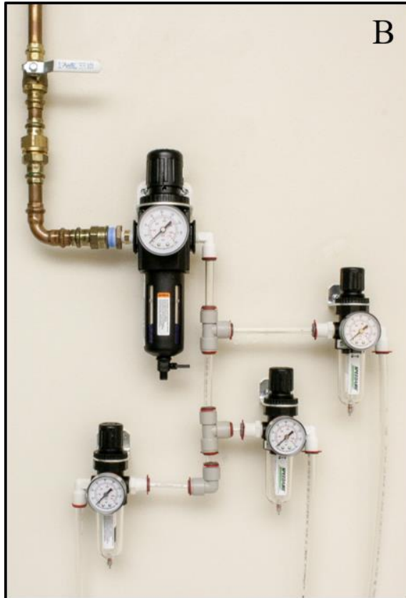
Figure 3B. Regulator setup for 3 FX-6000 FlexLinks
