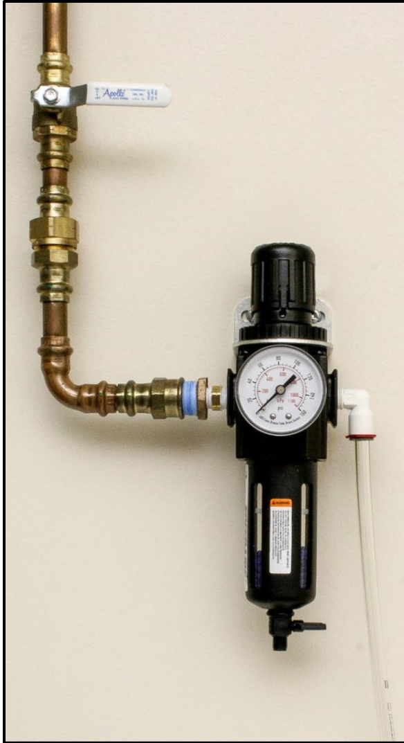
Figure 2. Single FX-6000 regulator setup
