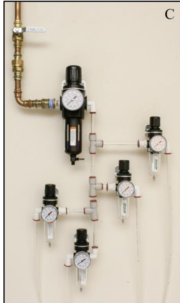
Figure 3C. Regulator setup for 4 FX-6000 FlexLinks
