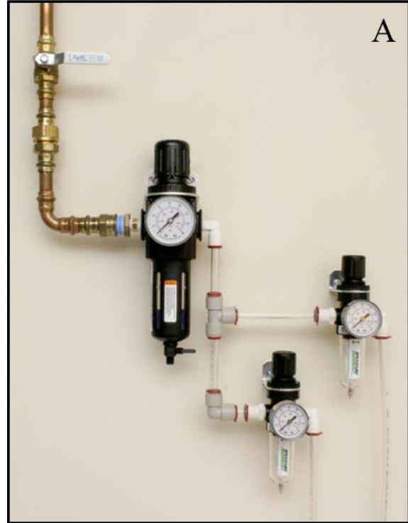
Figure 3A. Regulator setup for 2 FX-6000 FlexLinks
