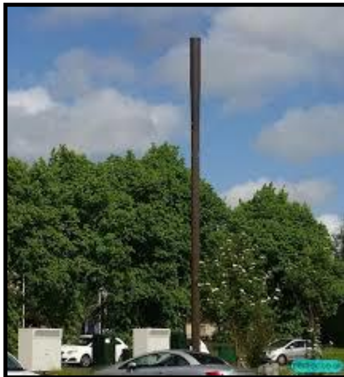
Figure 3 Typical 15m telegraph pole Mobile installation
