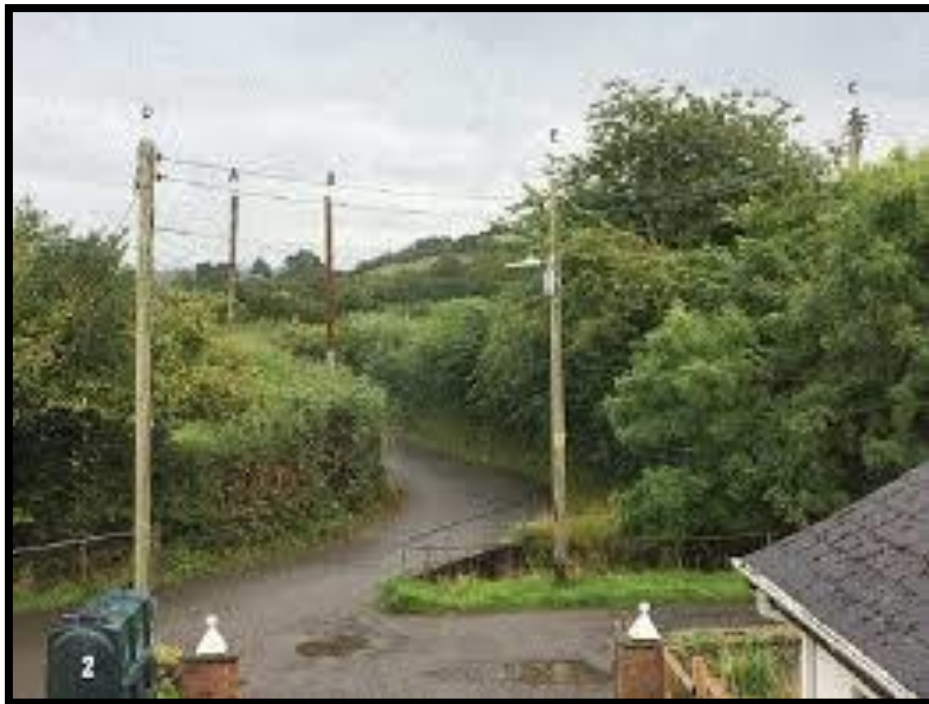
Figure 7 Example of Fixed Line Permitted Development Telegraph poles indicating increased number required
