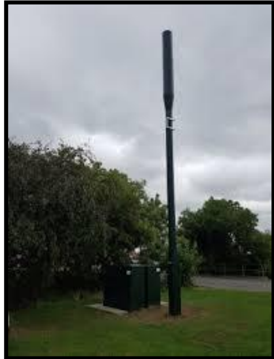
Figure 6 Existing installed smaller monopoles designs similar to a telegraph pole
