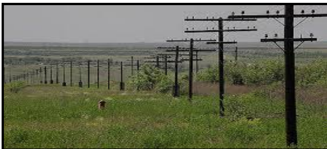
Figure 1 Indication of extent of telegraph pole deployment under a Reg 5
