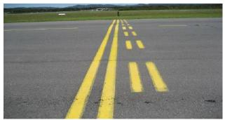
Runway Holding Points are provided at all Runway intersections. The Runway Holding Points consist of two solid yellow and two dashed yellow lines. The dashed lines are on runway side. With reference to the above picture, vehicles must hold on the left hand side of the two solid double yellow lines.
