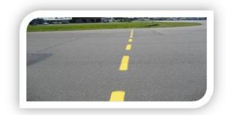
Intermediate Holding Points mark the intersection of Taxiways. For example; if you are given an instruction by Air Traffic Control to Hold Short of Alpha on Echo you would stop short of this type of marking.
