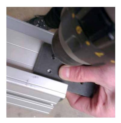
Drill holes using 6.2mm drill bit and countersink using a bit suitable for M6 Screws.
