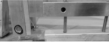
▲ ENSURE THERE IS ENOUGH CLEARANCE FOR THE B1 AND B2 PANEL SLOTS TO SLIDE BETWEEN THE WASHER/NUT AND THE A1 AND C1 PANELS.
