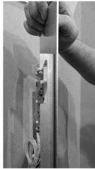
▲ SLIDE COP HOOKS OVER SCREWS MOUNTS.
