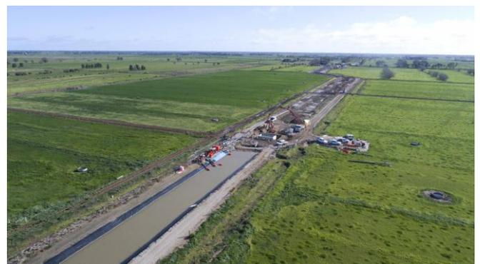
**Channel remediation:** Channel bank remodelling and lining is minimising water lost to seepage and leakage.
