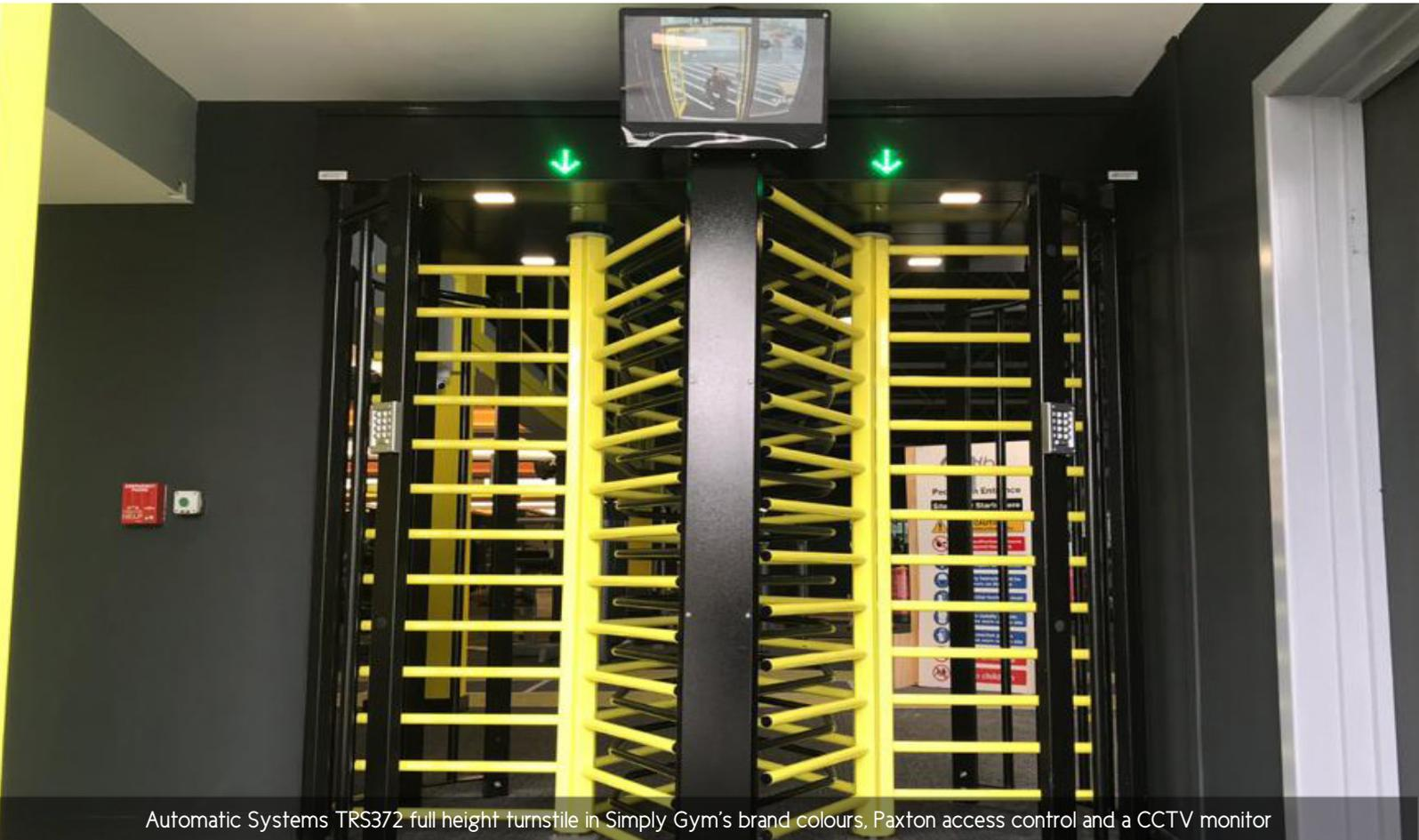
Automatic Systems TRS372 full height turnstile in Simply Gym's brand colours, Paxton access control and a CCTV monitor
