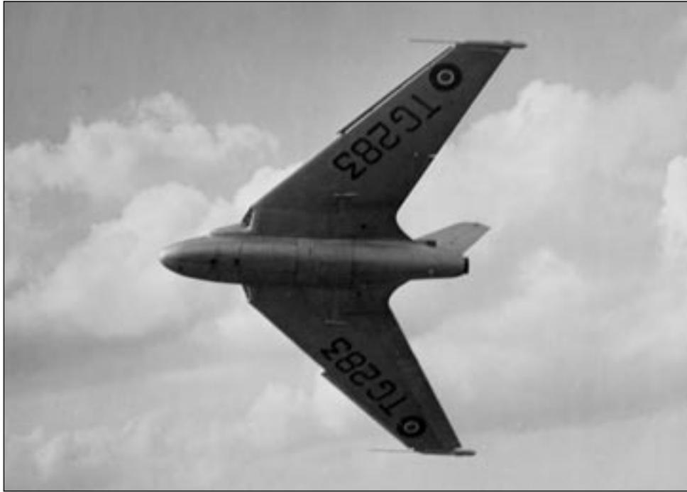
**Above:** The unique shape of TG/283 on a low pass, the leading edge slats clearly visible.
