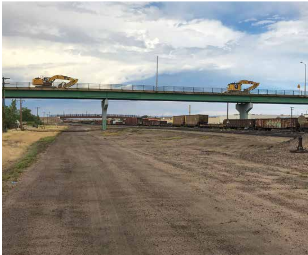
Excavators were used to assist in the demolition.
