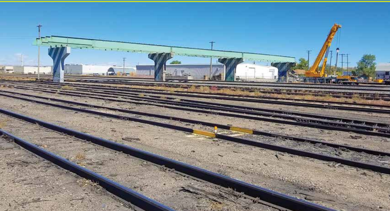
The bridge was demolished as part of a roadway relocation plan.
