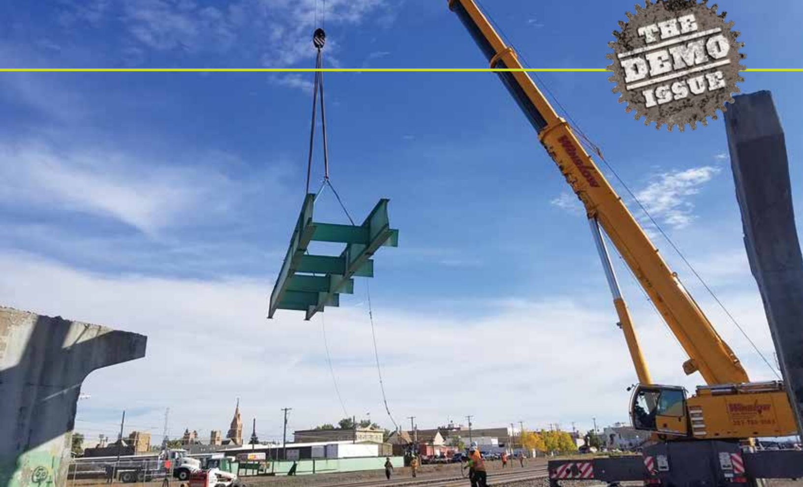
Cut sections were lifted out by crane.
