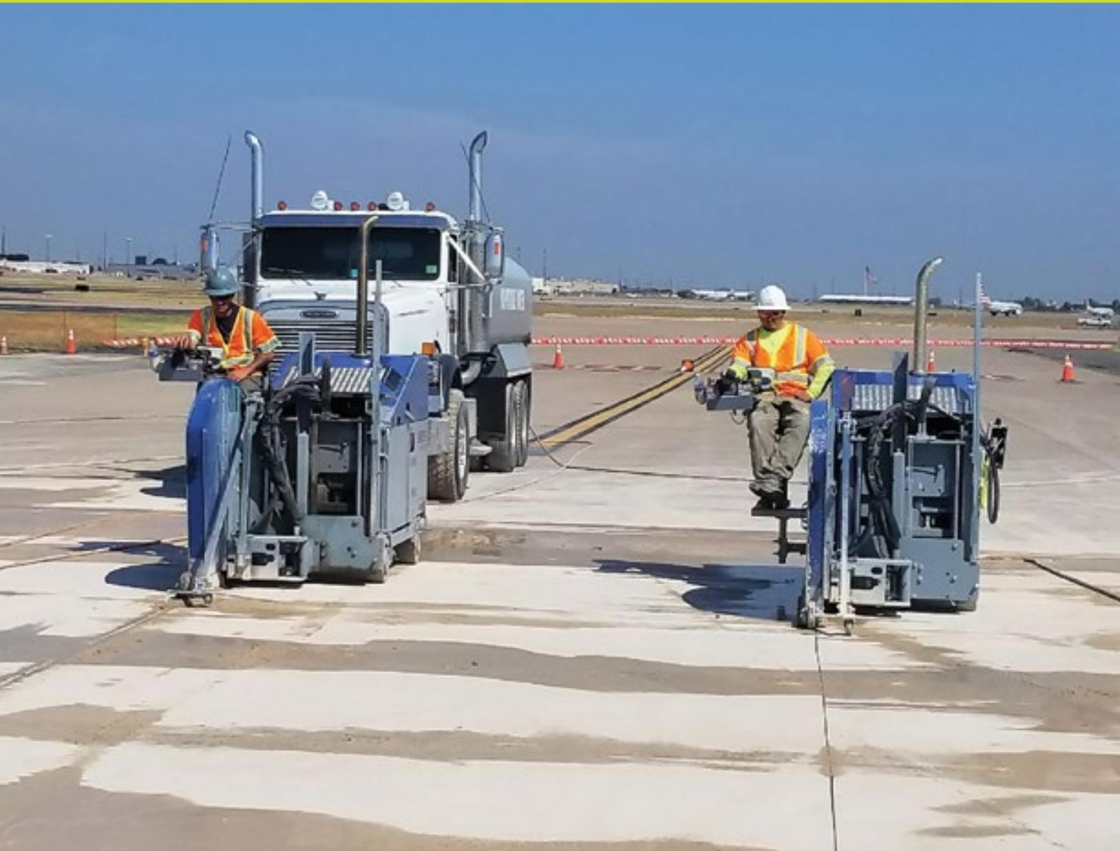
Dual rider saws from Lissmac make part of the over 115,000 square yards of cuts to remove the damaged portions of Runway 17C/35C at DFW.
