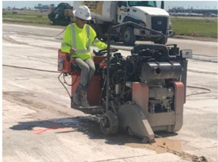
DDSC operator using a Husqvarna slab saw to make the cuts.
