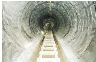
FIGURE 8 Field-seamed fabricated geomembrane panels used to create tunnel liner system (Geosynthetics.com).
