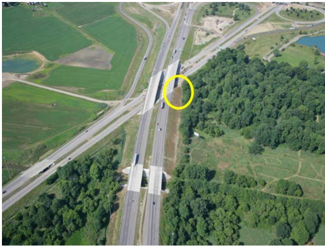
Fig. 5. Aerial view of I-71 Southbound between Stations 420 + 80 and 421 + 80 LT with I-76 crossing below it after remedial measures; circle shows the area prior to subject slope movement (photograph used with permission from ODOT)
