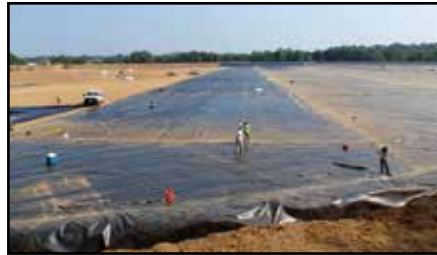
Geomembrane liner installation.
