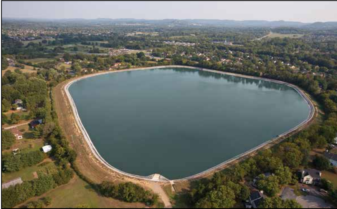
Aerial photo of the completed reservoir.
