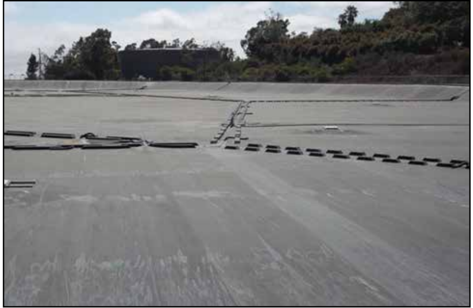
Figure 3. Floating cover rainwater collection troughs in service.
