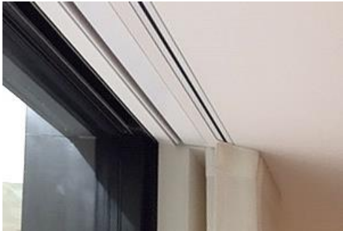
RT1F with SMB1F and SRB1F, installed in front of Blindspace box.
