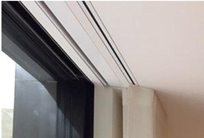
RT1F with QMB1F and QRB1F, installed in front of Blindspace box.
