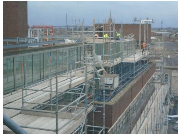
Figure 4: Window replacement programme
