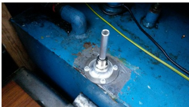
Dip Tube fitted as suction & return
