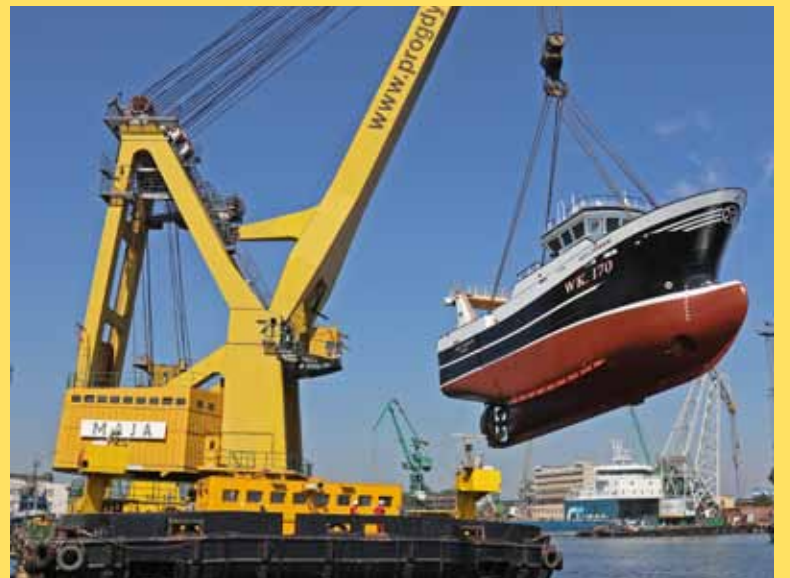
A large floating crane towers over Boy Andrew as the new whitefish vessel is lifted into the water.
