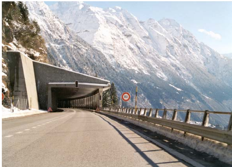
Fig. 2: Gallery Presella at the A13. The sensors are installed in the columns on the right.
